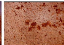
Rust embedded in the rock.
