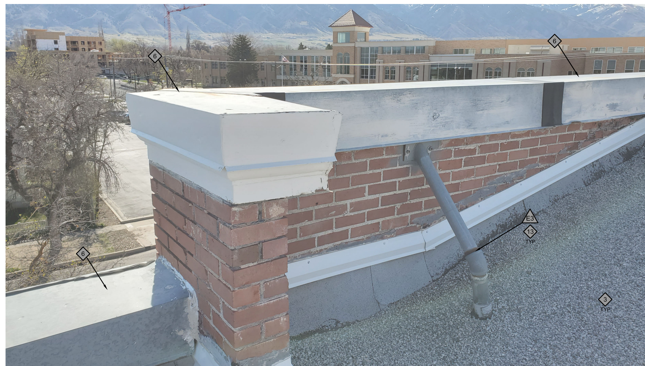
PHOTO: CHAPEL PARAPET AND BRACE
