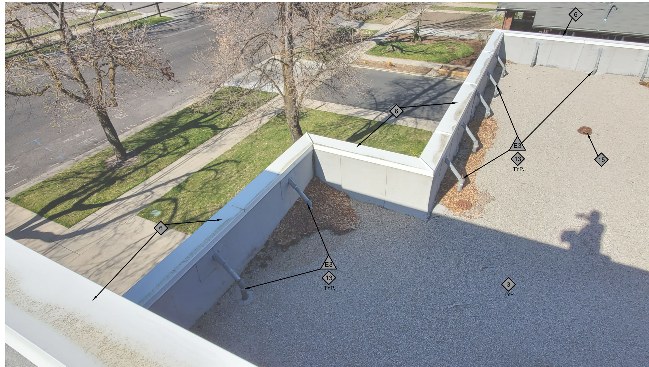
PHOTO: RELIEF SOCIETY ROOF (SOUTHWEST)
