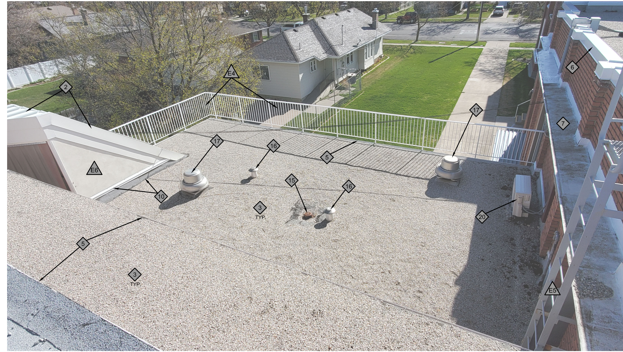
PHOTO: NORTH LOW ROOF
