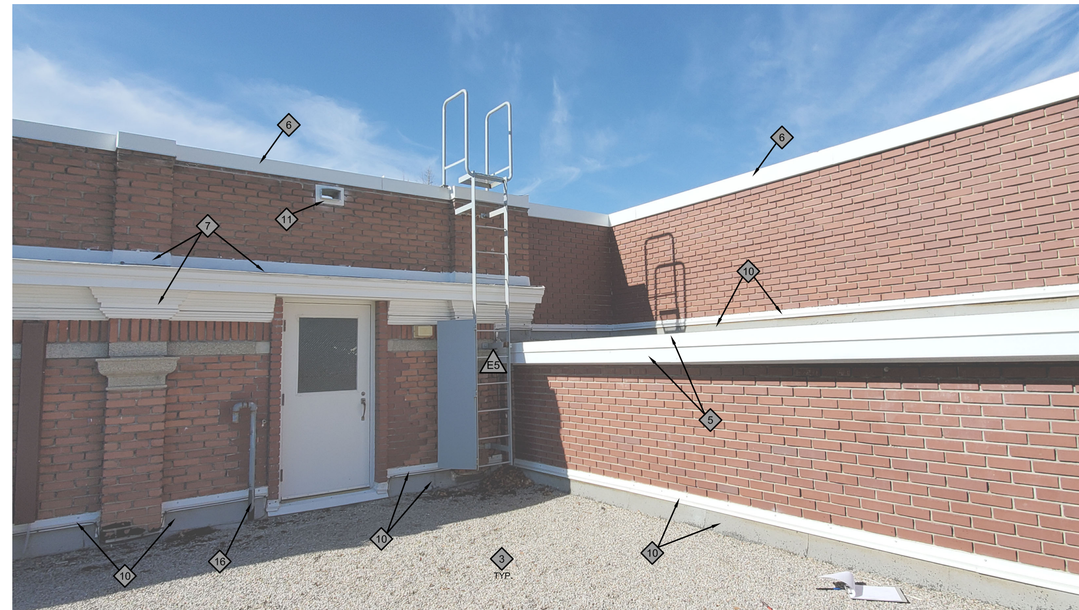
PHOTO: LOW NORTH ROOF LADDER AND DOOR
