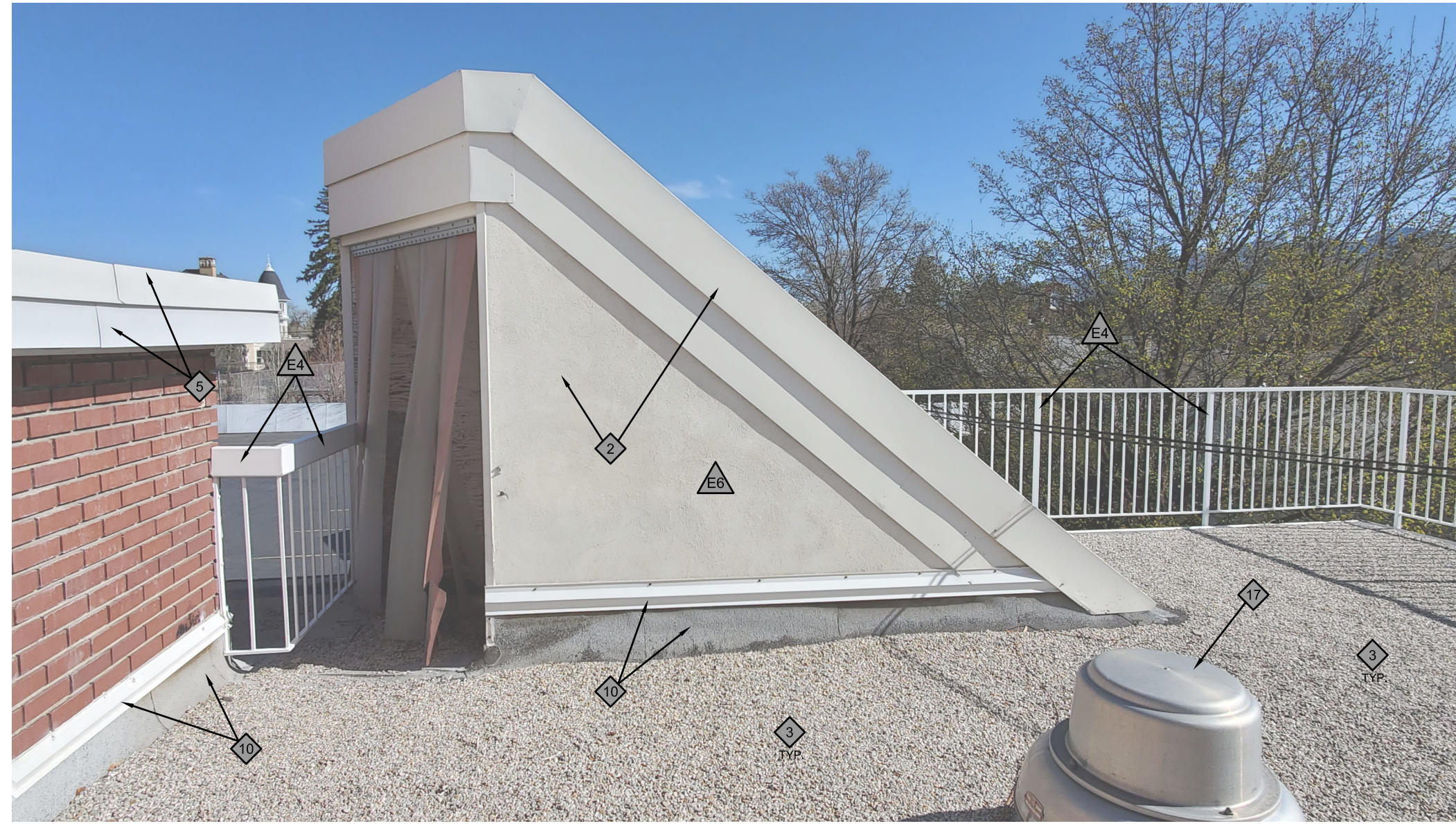
PHOTO: EXIT STAIR ON NORTH LOW ROOF
