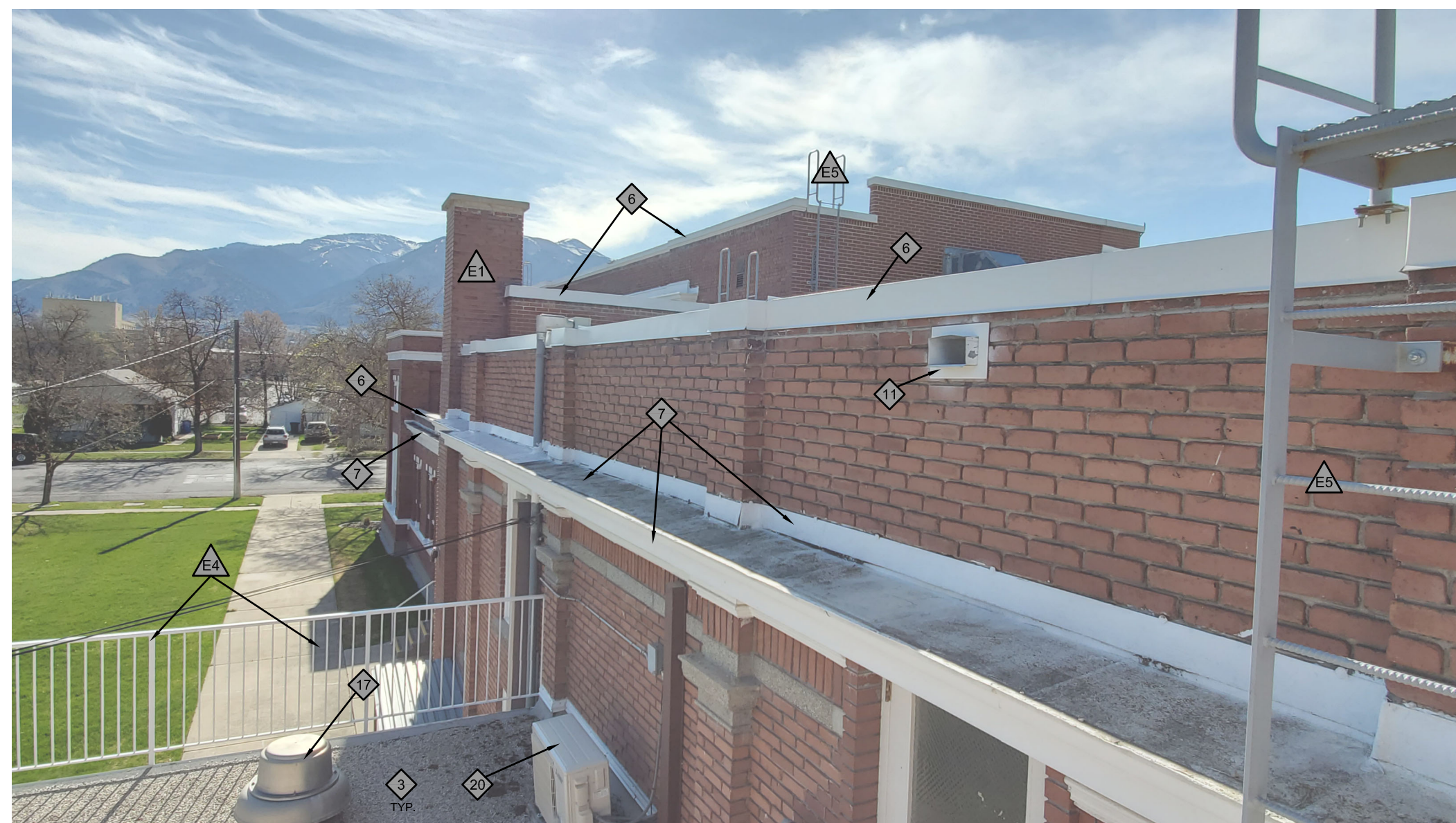
PHOTO: NORTH INTERMEDIATE ROOF
