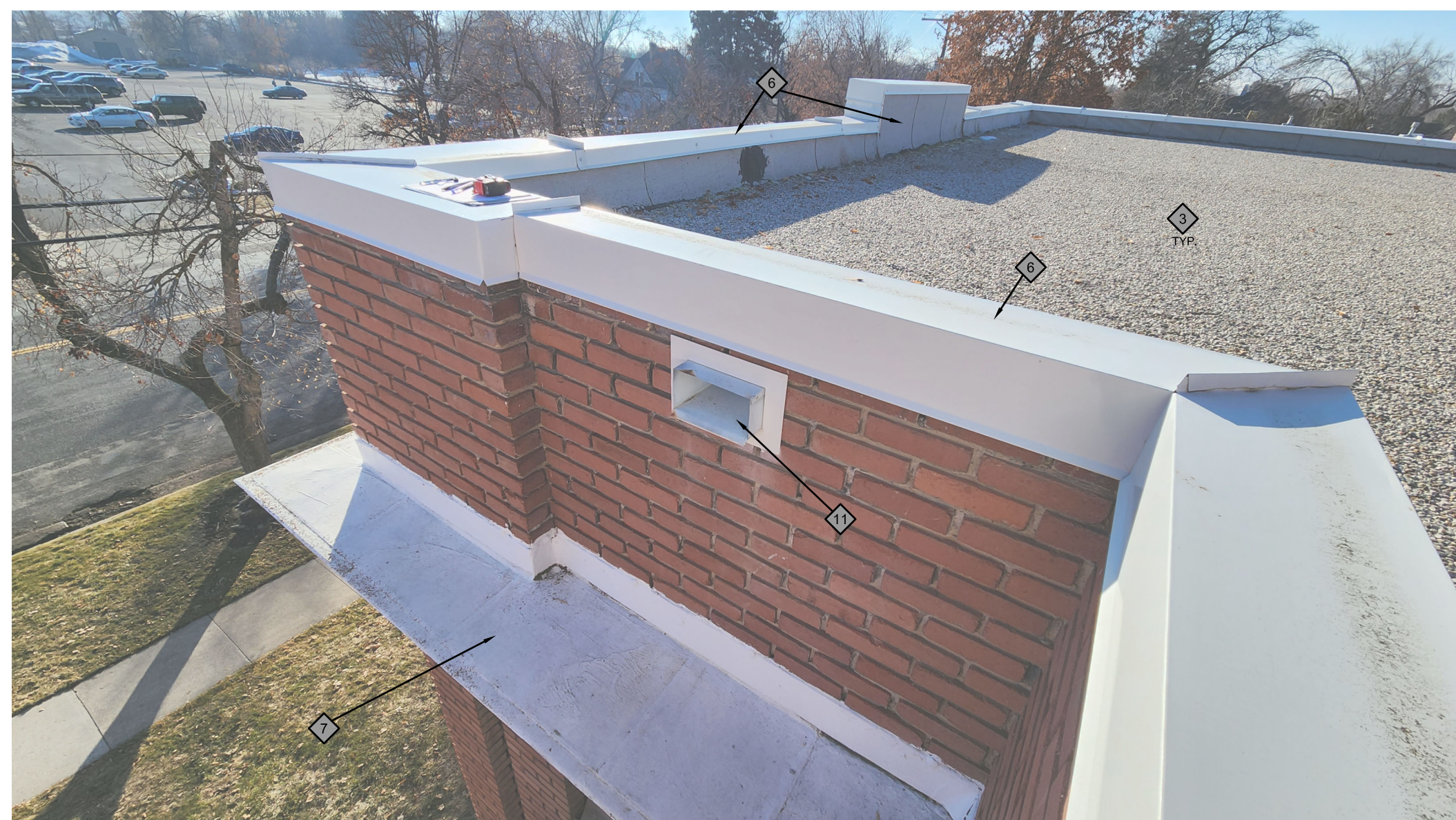
PHOTO: SCUPPER AND METAL CAPS
