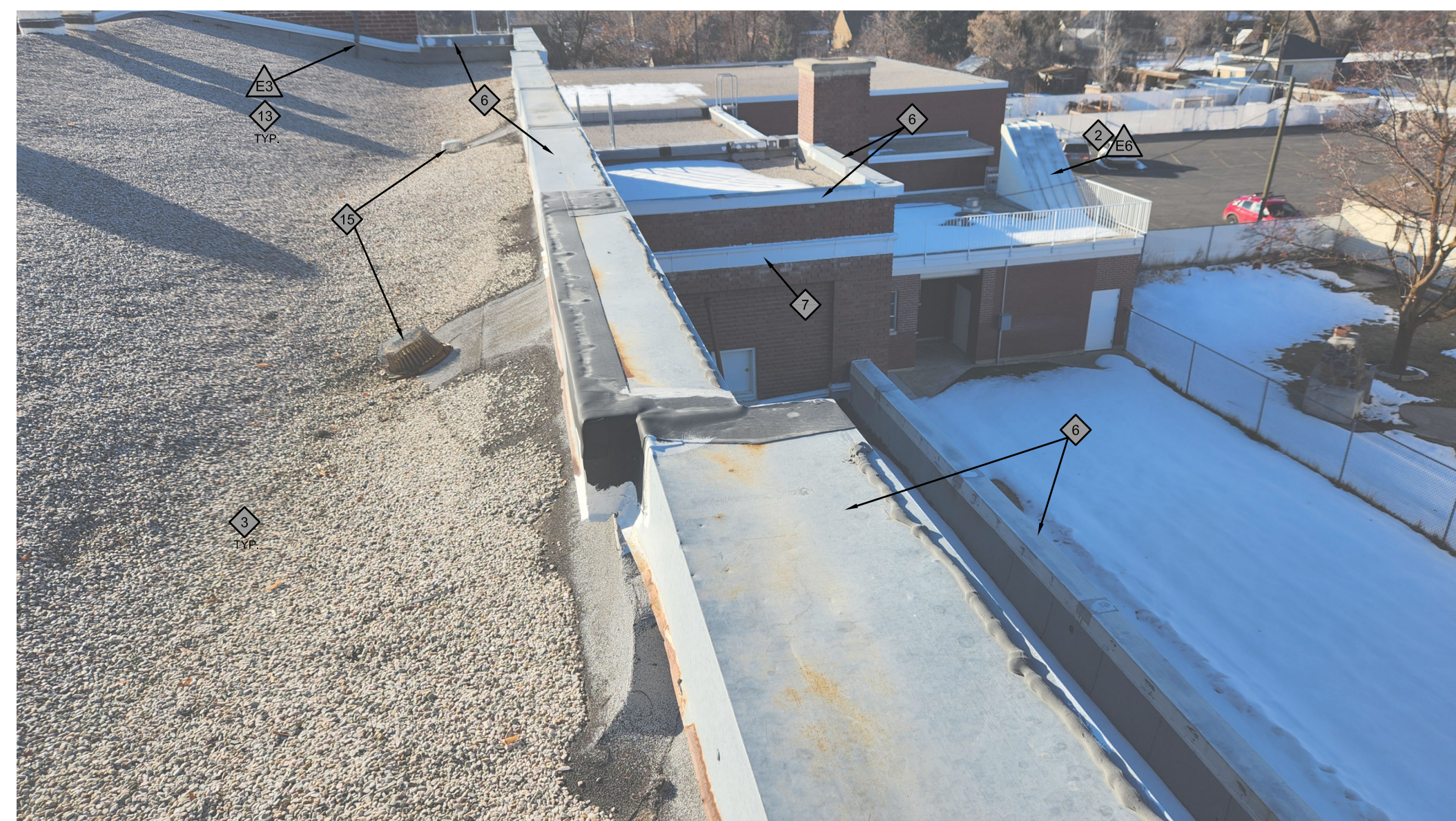
PHOTO: PARAPET CAPS
