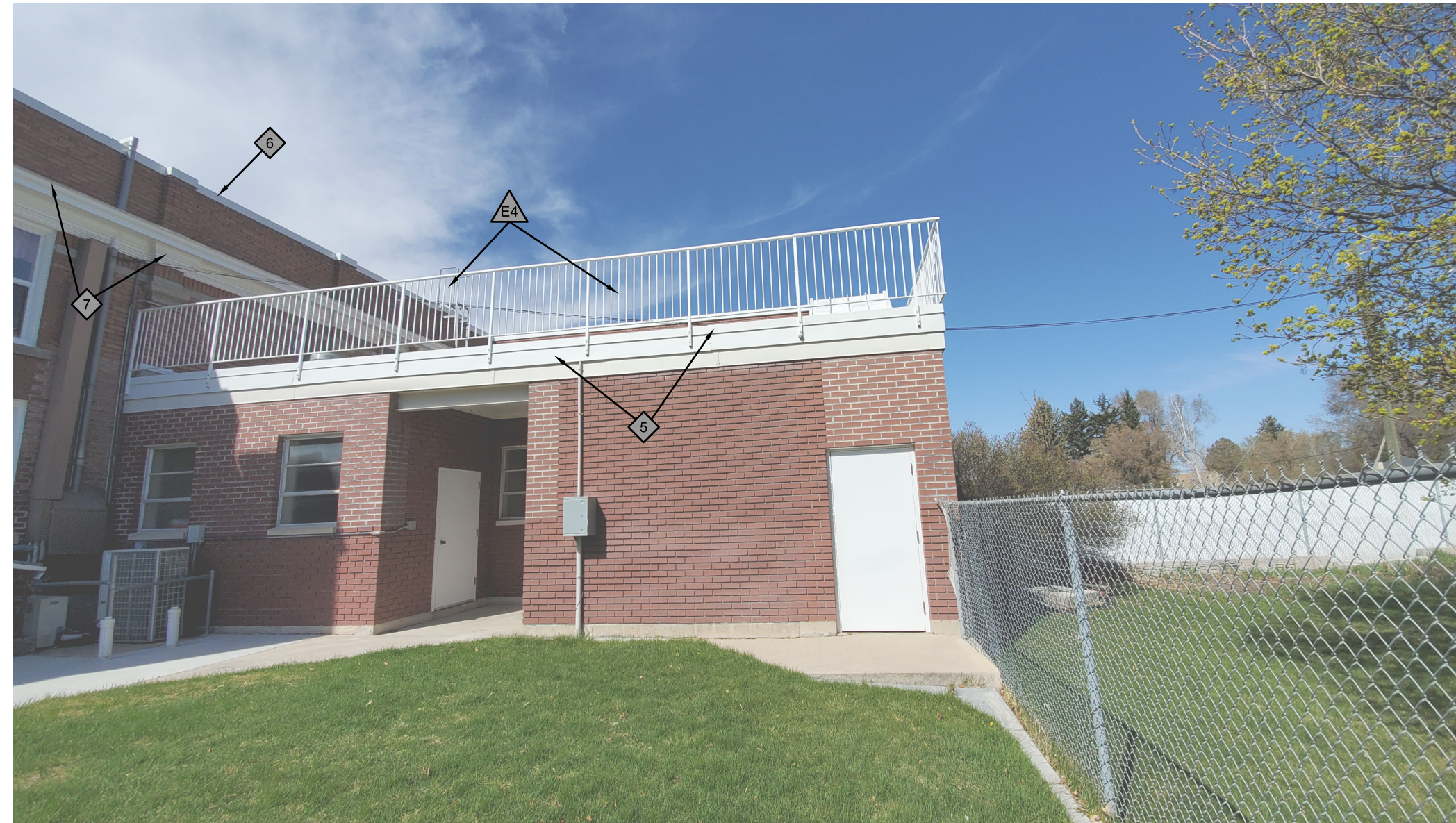
PHOTO: NORTH LOW ROOF RAILING
