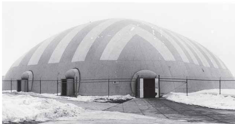
"The Bettendorf Bubble breathed a last beleaguered breath when Jim Kennedy unplugged the air supply," according to the June 28, 1978 Bettendorf News. Kennedy purchased the bubble and planned to use it for something, somewhere, according to photographer Ron Burbridge.
