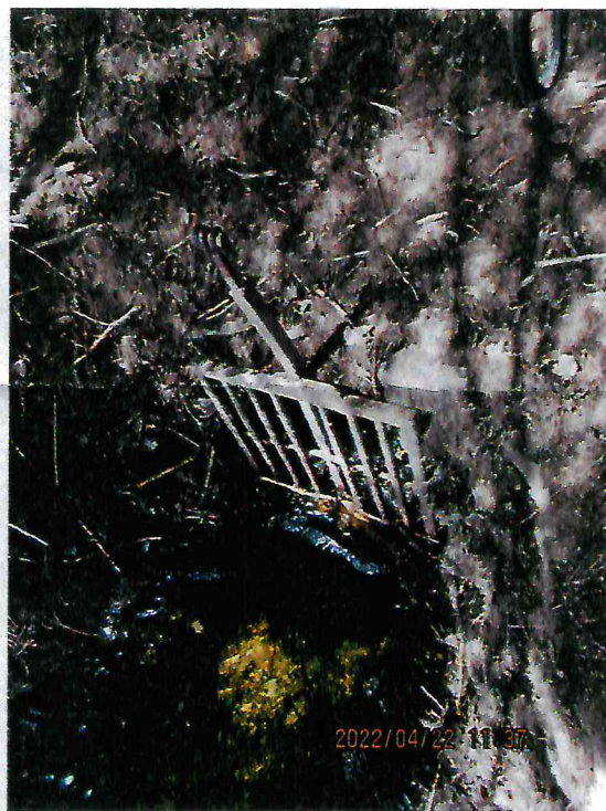
Photo 2. Primary spillway culvert inlet and grate.
