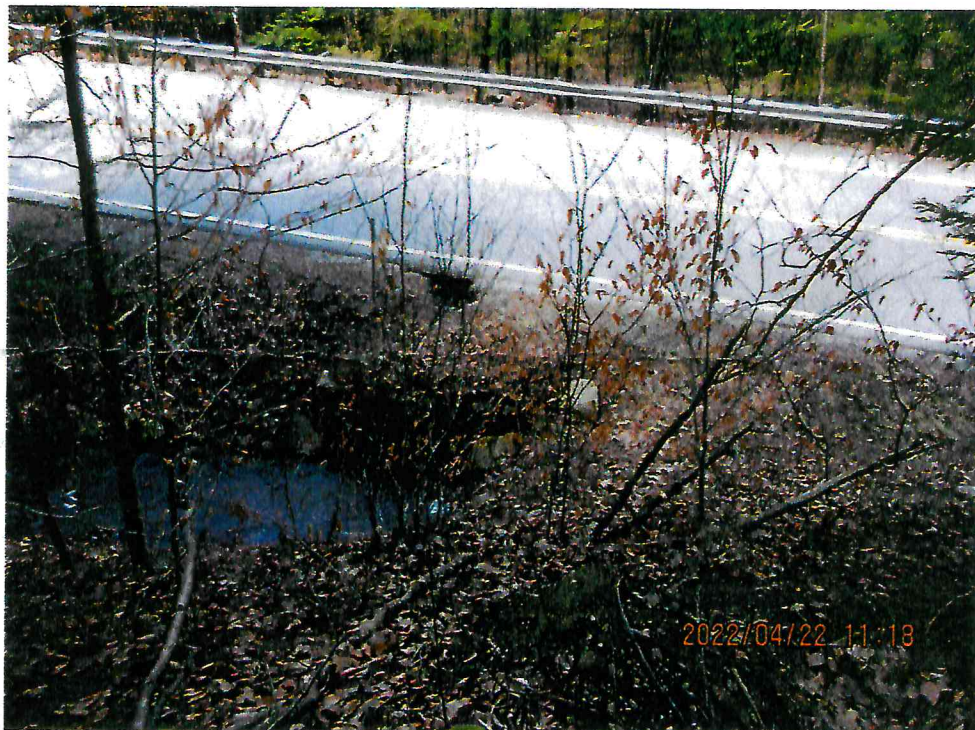
Photo 6. Downstream Route 63 culvert crossing upstream inlet.
