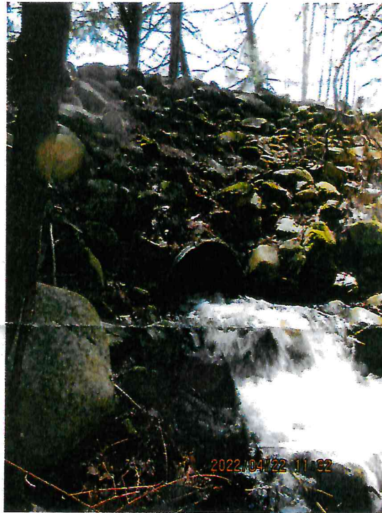
Photo 5. Downstream spillway outlet and discharge area.
