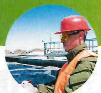
Water/wastewater treatment facilities
