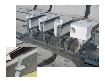
Arecon designs and installs vapor intrusion mitigation systems.
