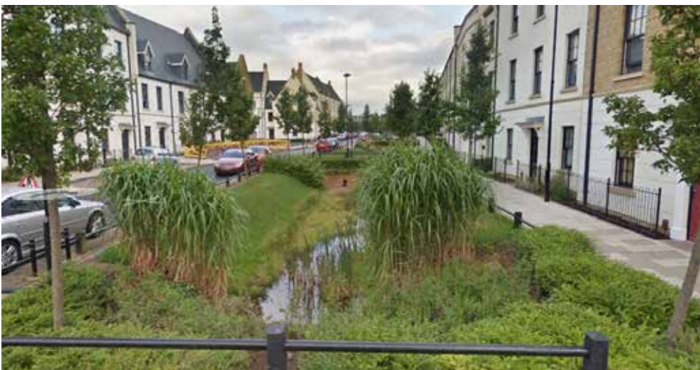
This 'ditch' in a built up area is a functional drainage channel, a wildlife corridor and an attractive addition to the street. Photo: Google
