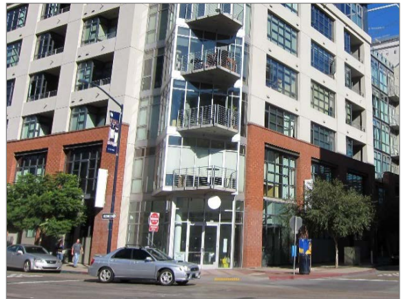
An identifiable change in materials and articulation defines the base of multi-story buildings.
