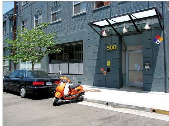
A simple canopy, lighting, and recessed door lead pedestrians to the primary entrance of a building.
