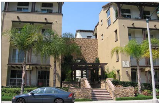
Stairs from the sidewalk leading up to the common entry of a residential building invite pedestrian access.
