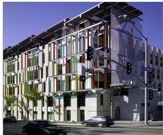
An external skin made of colored glass panels adds visual interest to concrete parking structures.
