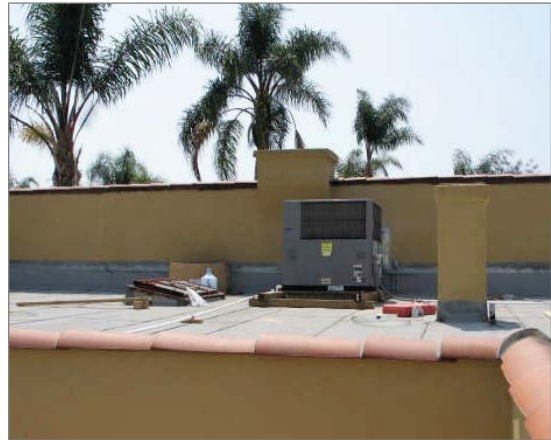
Rooftop mechanical equipment should be placed behind a parapet to screen it from public view.
