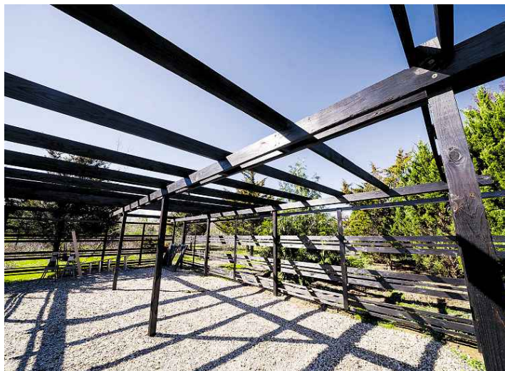
An eye-catching entrance pavilion and adjoining overhead structure have been treated in the Japanese technique of shou sugi ban .
