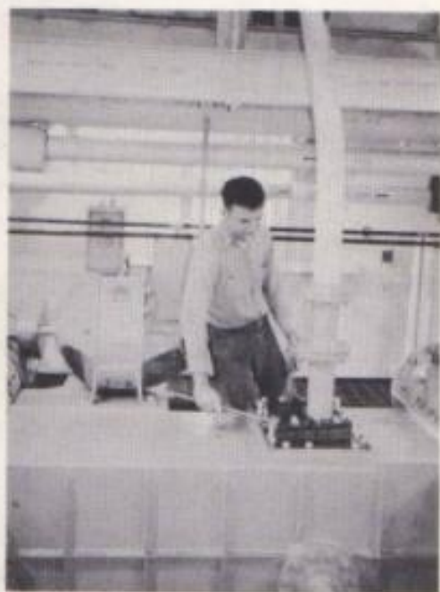
Inspection of main reduction gear.
