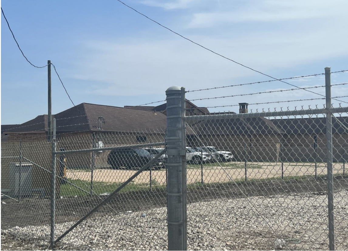
Figure 7 VisionQuest facility facing county-used field
