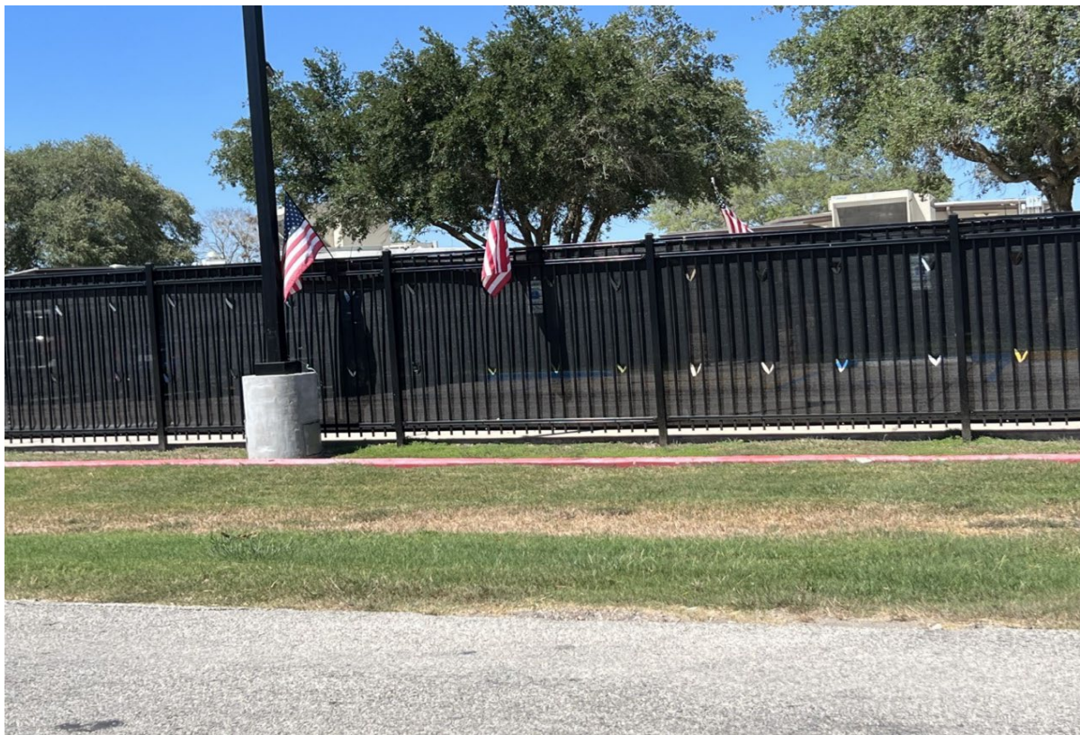
Figure 4 Endeavors Eagle Lake facility fence faces residential street
