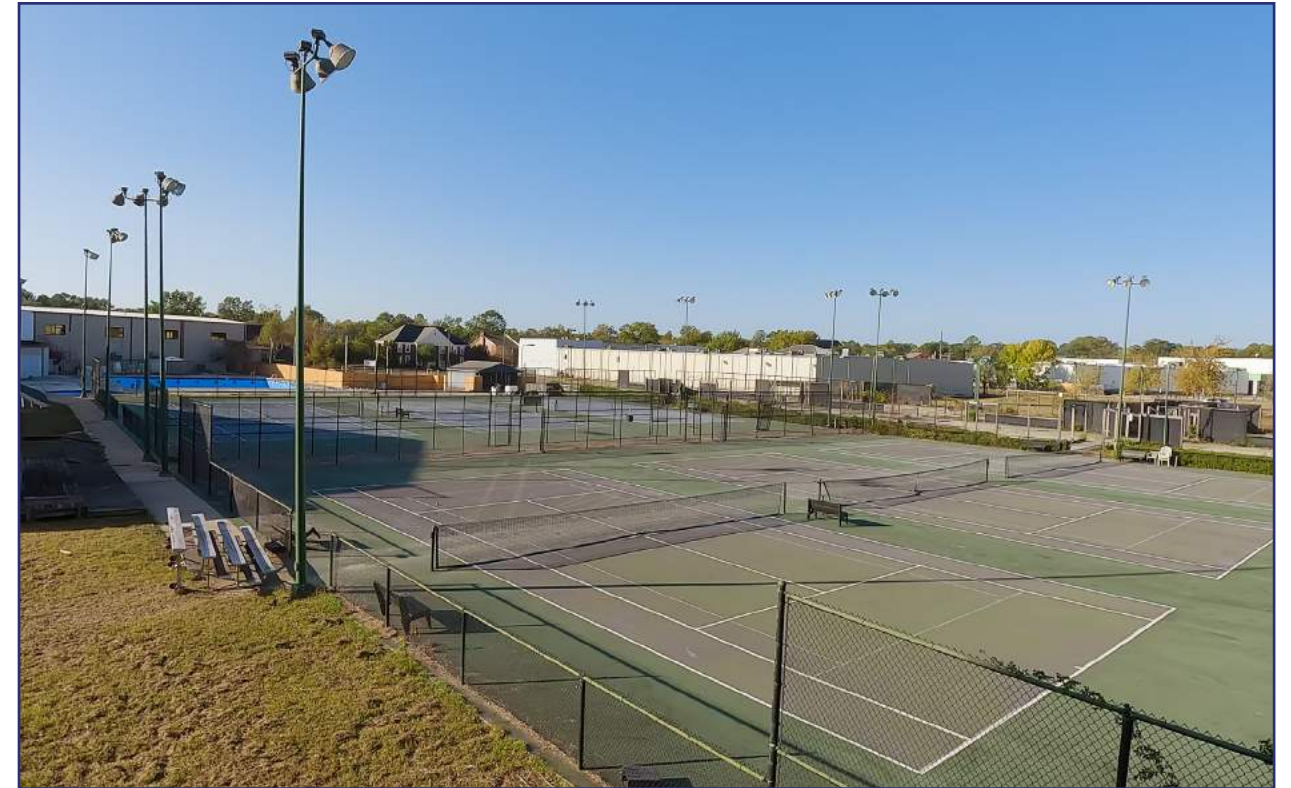
Outdoor Hard-Surface Tennis Courts
