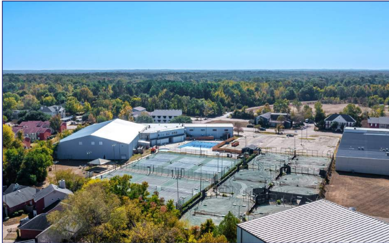
North Aerial View
