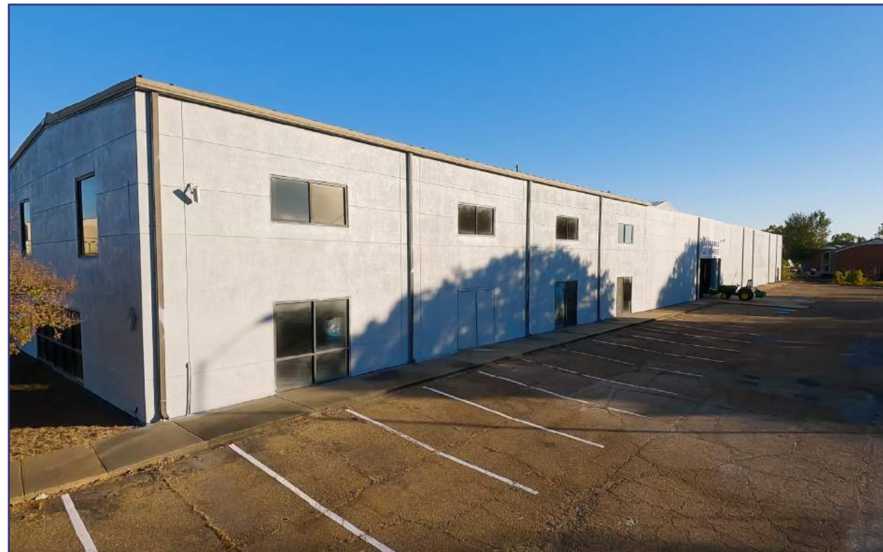
South Parking Lot and exterior facade
