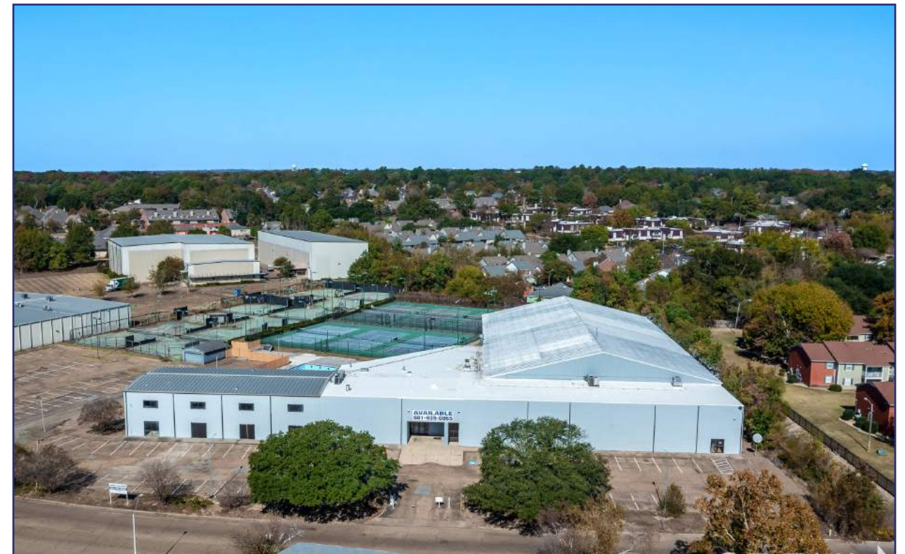
Front of Building from Northtown Drive
