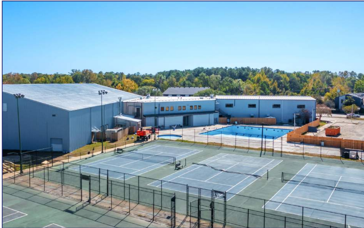
Outdoor Hard-Surface Tennis Courts
