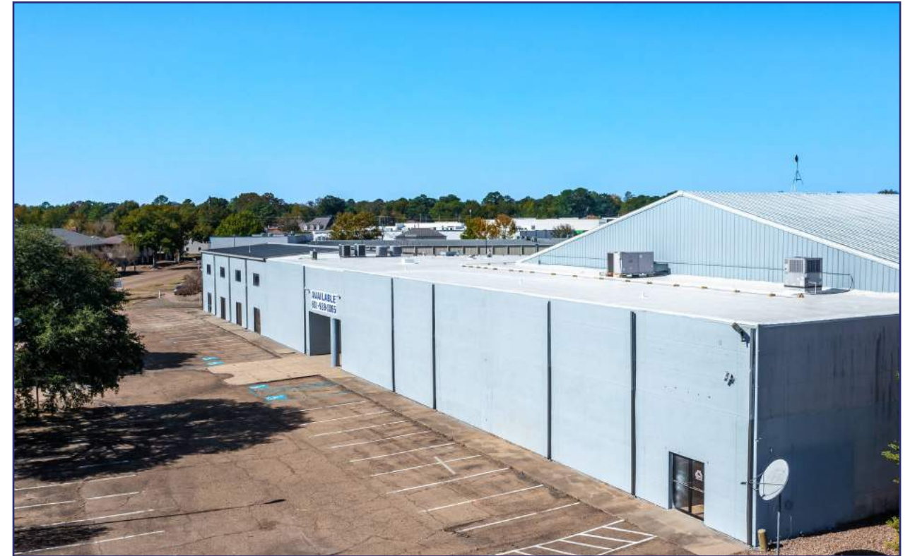
Southwest Aerial of Building
