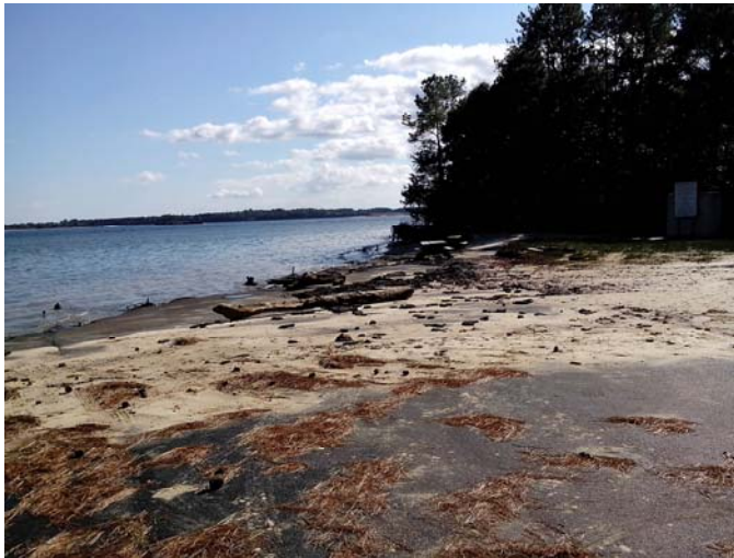
Erosion of beach after October storm
