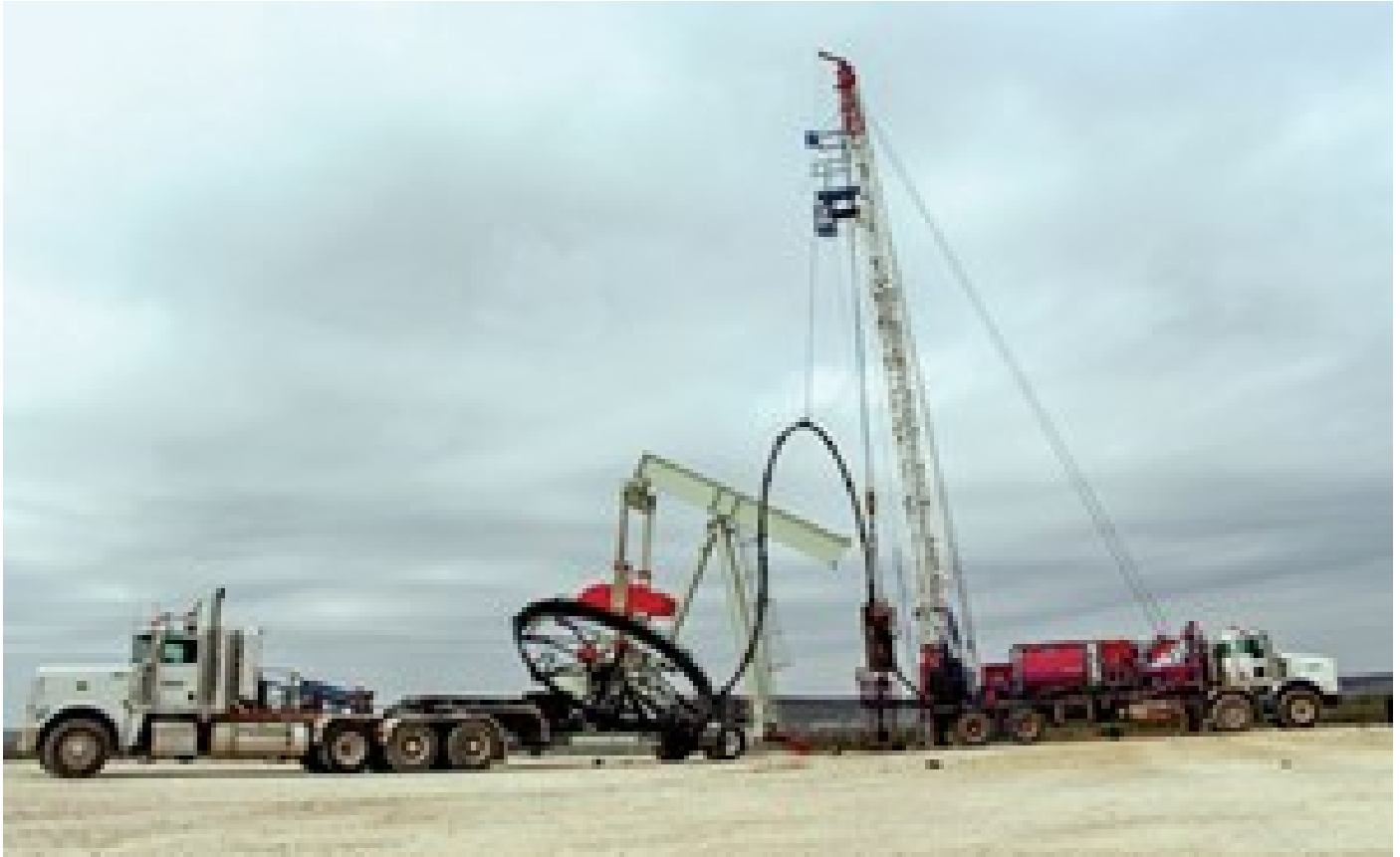
Fig. 3. A LPS crew replacing a conventional sucker rod string with coiled rod.
