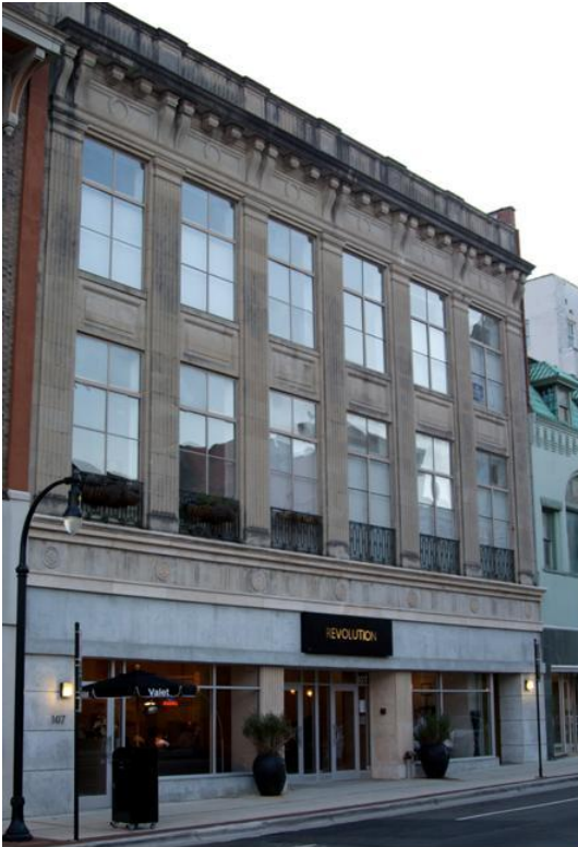
Storefront: Aluminum with clear, anodized finish. Transparent window glass. Two entry doors for Commercial Unit, separated by two glass panels. Both doors swing outward. Entry alcove into Residential Units has single door swinging outward with same clear, anodized finish.
