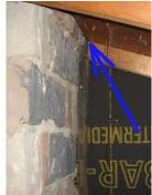
17. Attached Garage Attic Sheathing: Plywood - Water stains and slight damage present, Areas of sheathing have been repaired
