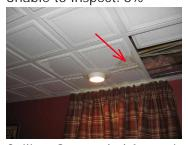
Acceptable Ceiling: Suspended Acoustical System - Evidence of past water staining
