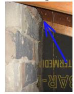
Marginal Sheathing: Plywood - Water stains and slight damage present, Areas of sheathing have been repaired
