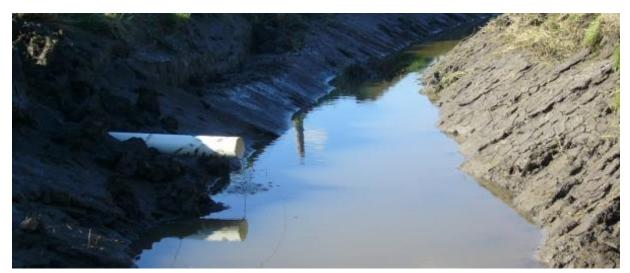
When the water table in the soil is higher than the polydrains, water flows into the holes of the corrugated polydrain. This lowers the water table to the depth of the drains over the course of several days. Subsurface drains allow excess water to leave the field, but once the water table has been lowered to the elevation of the drains, no more water flows through the drains.
