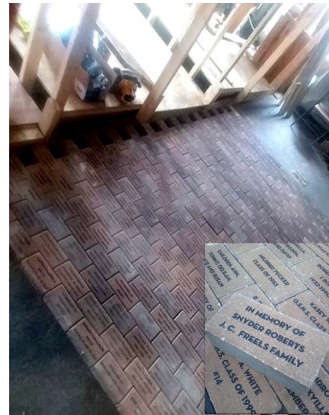
Streetscape Under Construction
