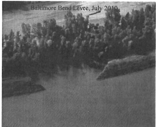
Baltimore Bend Levee, July 2010
