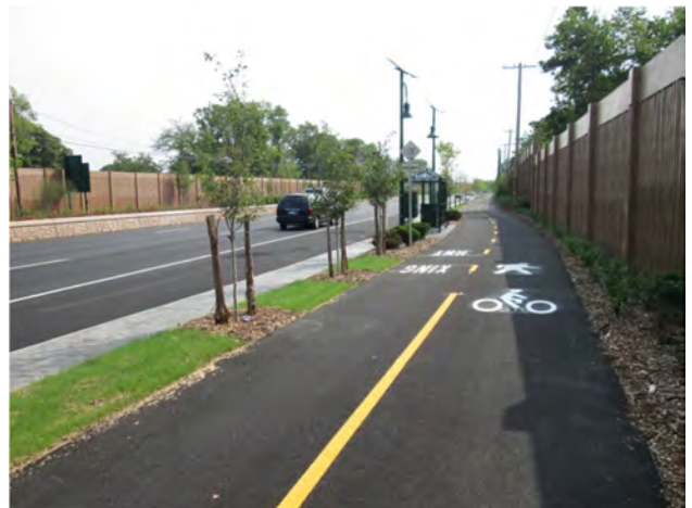
Photo of completed section of NY 347 in Hauppauge/Smithtown. NYSDOT had developed this Complete Streets concept for the entire length of NY 347, from Hauppauge to Mt. Sinai in the Towns of Smithtown and Brookhaven. The noise walls are constructed in residential areas that abut NY 347. Improvements include a shared-use path along the south side of the roadway and bus stop shelters. Source: Google Earth
