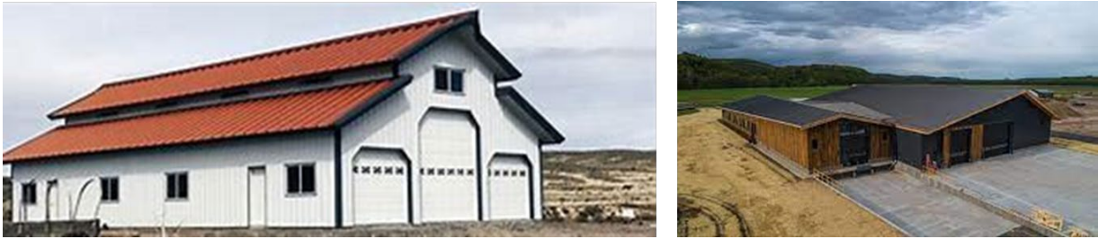
Figure 3.3-4. Example of light industrial buildings that are compatible with surrounding agricultural landscape
