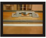
Examples of Pot Metal Hardware after Use. Paint can Scrape Away and Expose Raw Metals and Dust!
