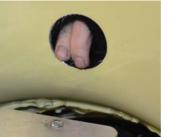
It's no place in France, but there's definitely a hole in the wall! We'll clean up the rough edges before moving along to install the grommet. These screw-on grommets are a staple around the shop. They come in a multitude of sizes, are aesthetically pleasing, and can be trimmed to fit however much we
