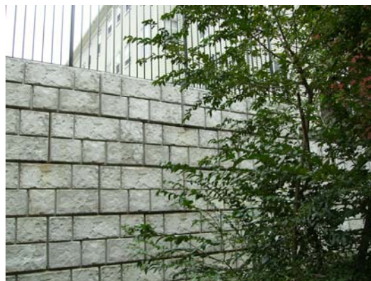
Quarry Cut Face without Cap
