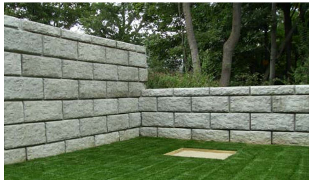
Rough Stone Face with 1 Foot Rough Stone Cap*
