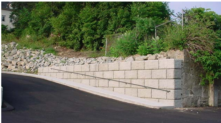
Railing Attached to Wall—Functional and Aesthetically Pleasing
