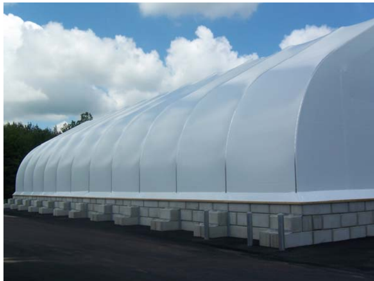
Built-in buttress system strengthens side wall
