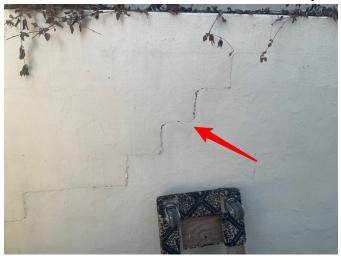
**18:** The rear CMU yard wall, behind the pool equipment, can be easily moved, and should be evaluated by a masonry contractor.
