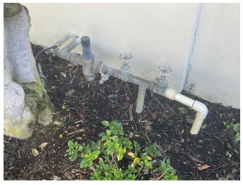
**83:** The main shut off valve consists of a gate valve rather than the ball valve. Gate valves will deteriorate, rust, and freeze up over time. We recommend replacement as an upgrade in the near term.
