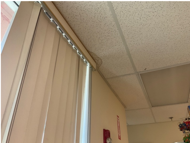
Over main entry doors
