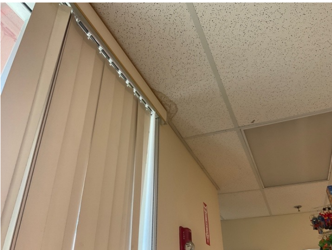
Over main entry doors
