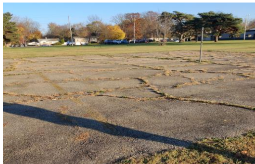
Unused pavement north of Wainwright School.
