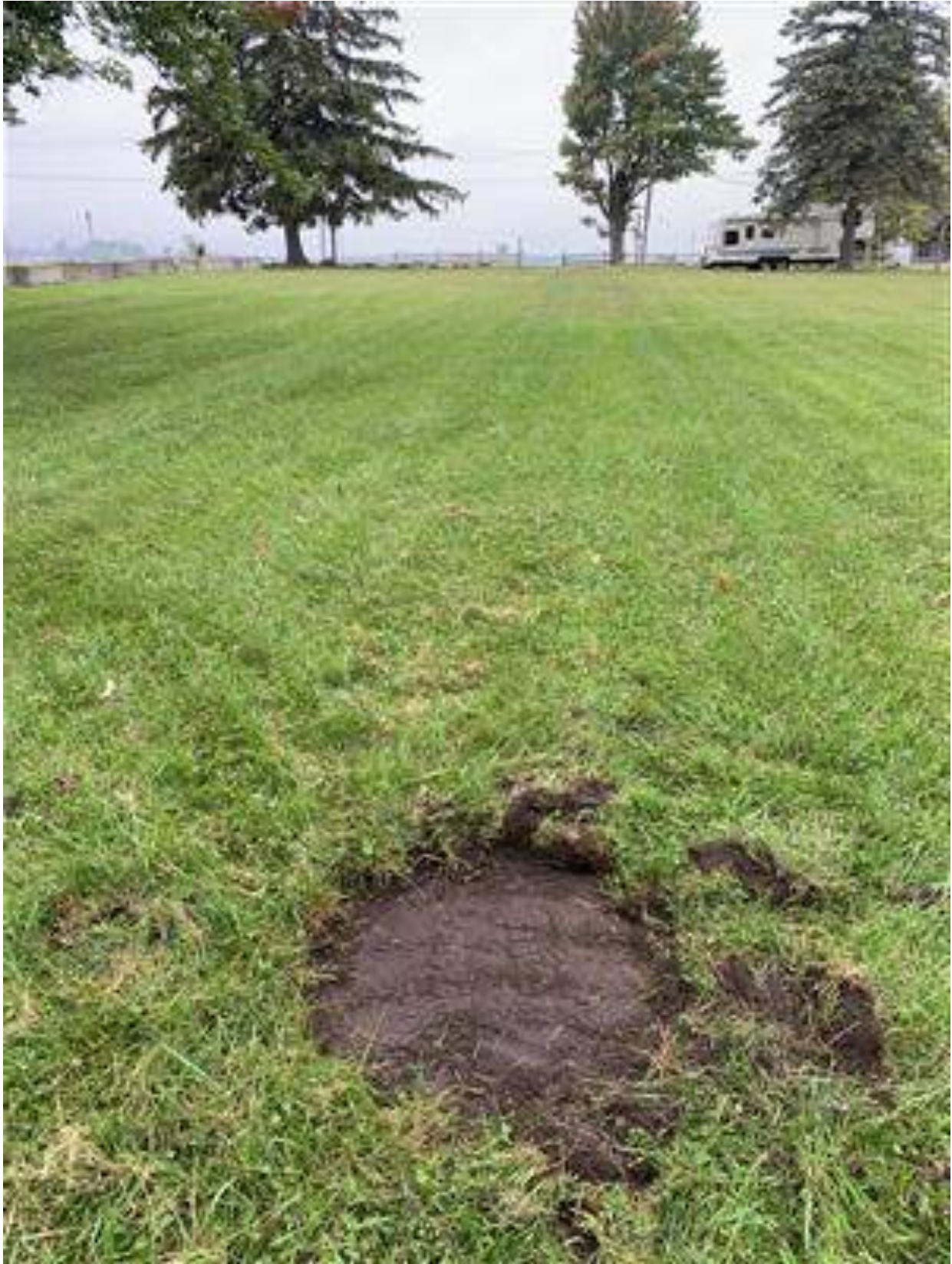
One of the Manholes to be Rehabilitated
