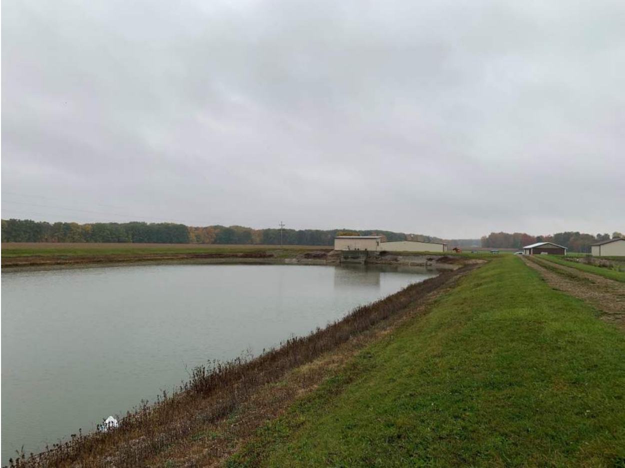
Lagoon and Maintenance Building at WWTP
