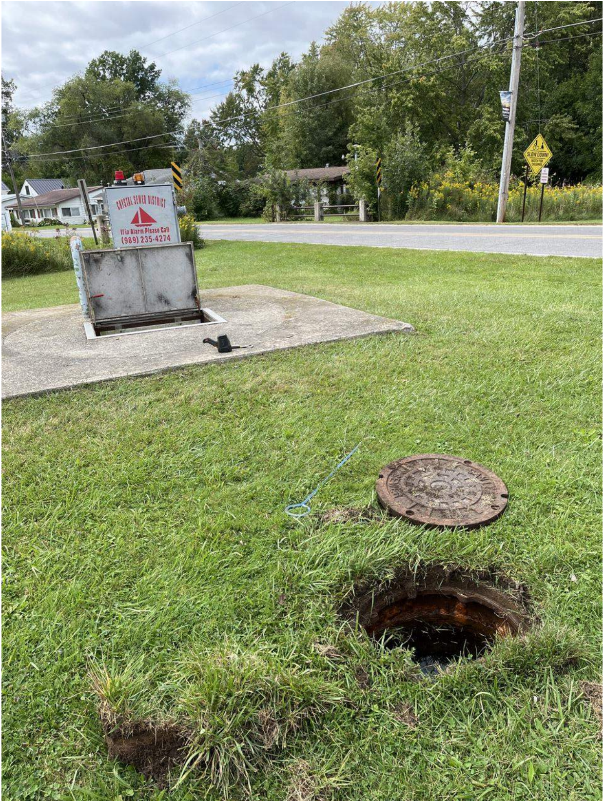
One of the Lift Station Valve Chambers to be Rehabilitated
