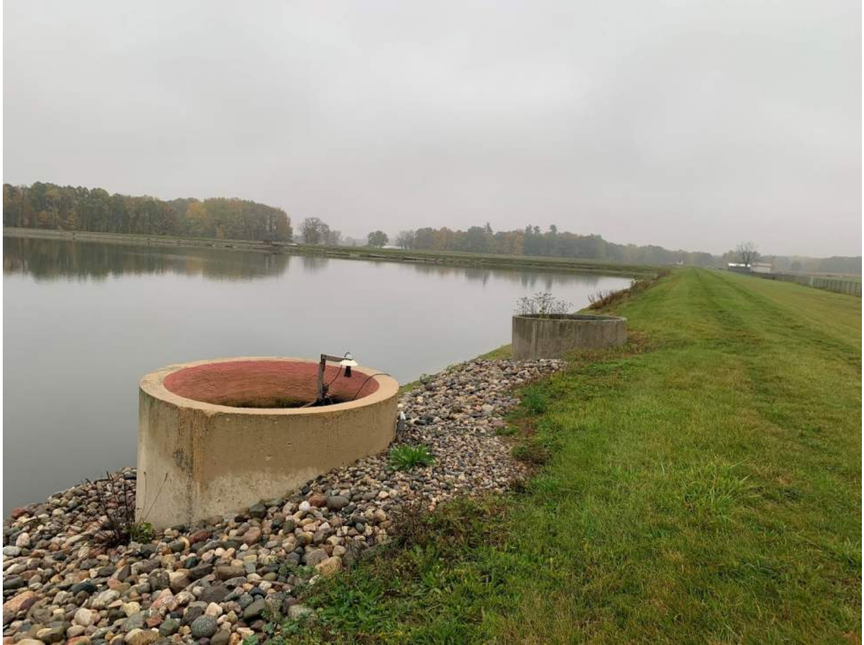
Examples of Structures to be Rehabilitated at WWTP
