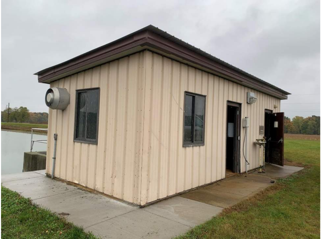
Irrigation Building at WWTP – To be Reconstructed
