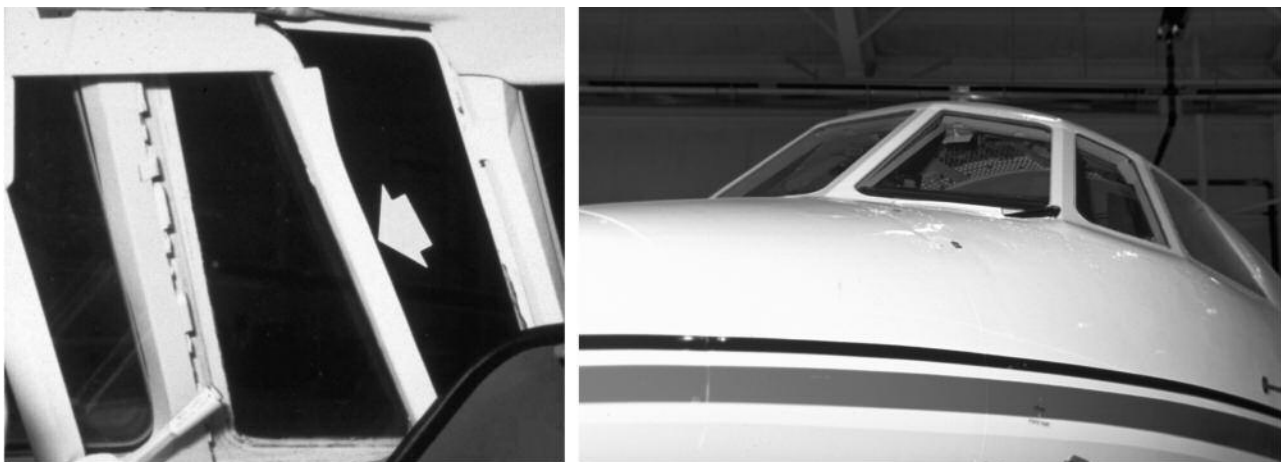
SLIDING WINDOW PANEL SEEN FROM INSIDE
