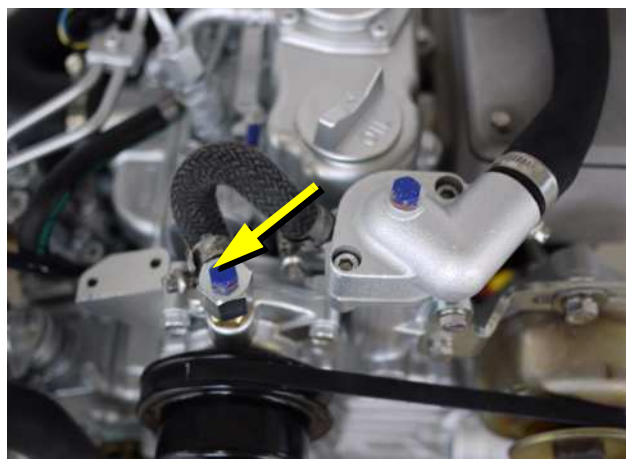
Fig. 3.3.2-5: Ventilation Screw Fresh Water Cooling Pump
