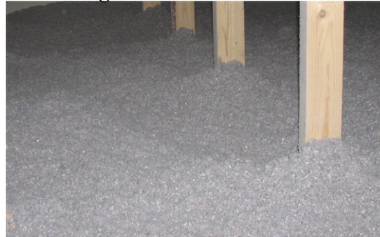
The ceilings and walls of your home are full of odd shaped cavities and obstacles like plumbing, air ducts and wiring. For your insulation to work properly, it must completely fill around these obstructions. **ThermShield** is a custom-fit insulation for your home.
