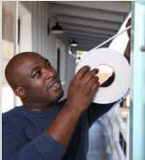
**Felt** This is the most affordable weather stripping option, but the least durable. A synthetic blend of fabric or wool is installed around a door or window sash.
