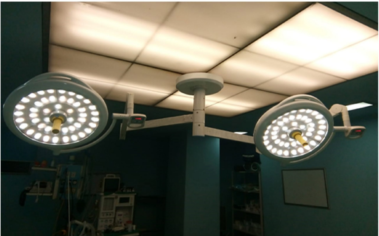
Low Height OT solution where clearance height is between 8ft and 9ft
