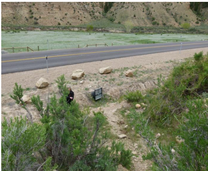
Figure 8. Below the panel looking back towards the valley floor, is a large culvert that when open diverts the water under the modern road bed.
