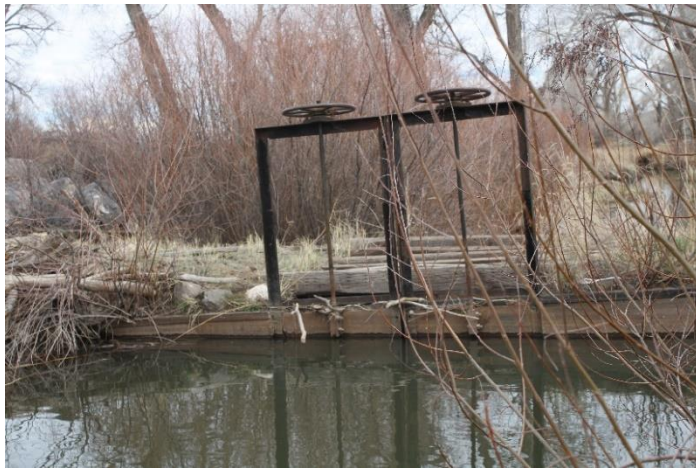
Headgate looking downstream
