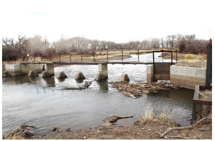
Headgate and diversion dam
