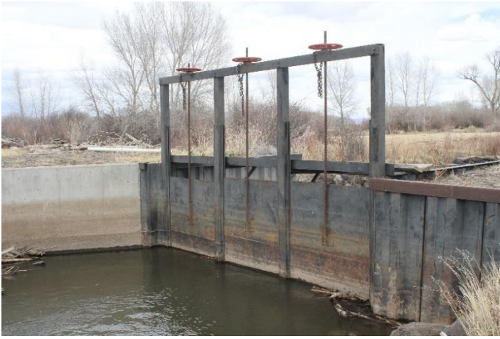
Headgate looking downstream
