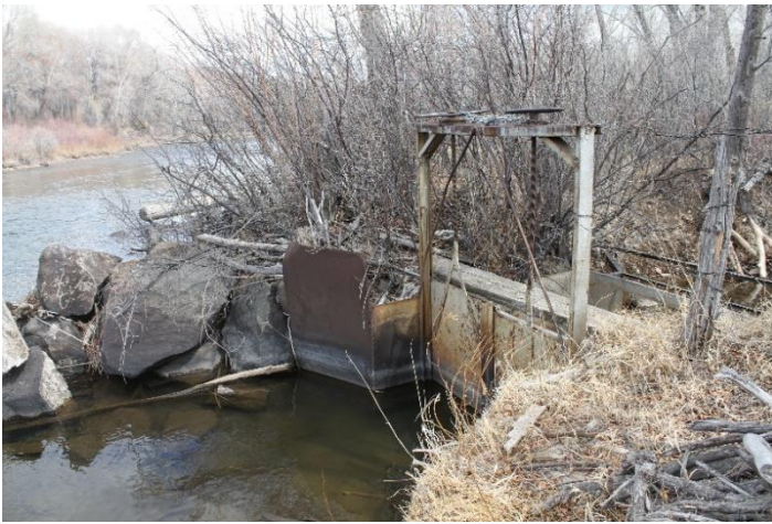
Headgate looking downstream
