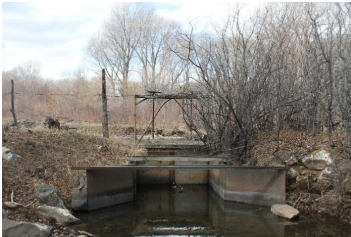
Bank stabilization upstream of headgate
