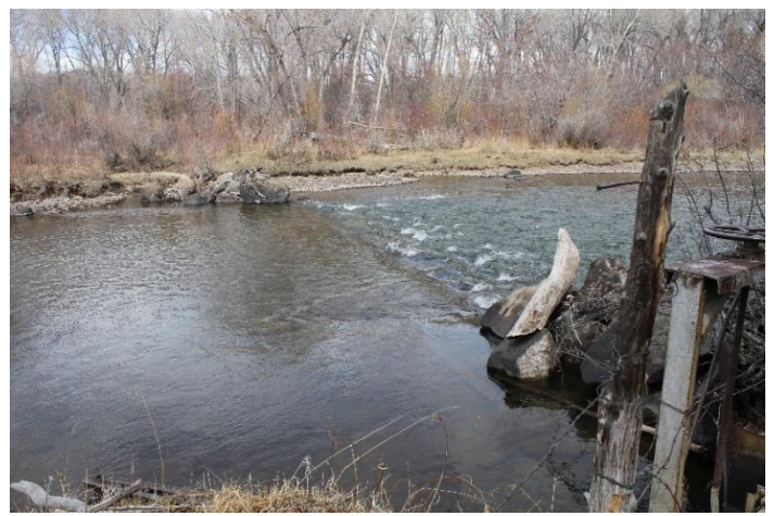
Headgate and diversion dam
