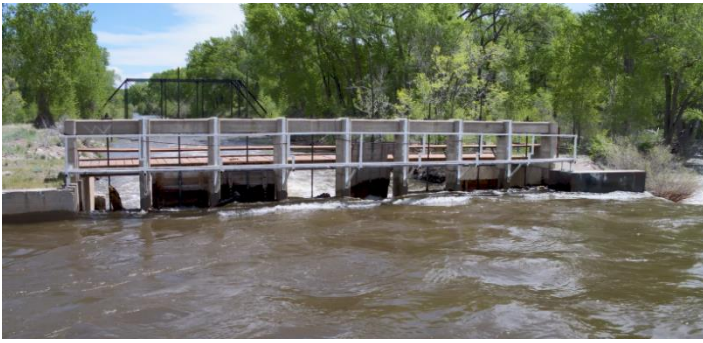
Headgate for North Channel Rio Grande looking downstream
