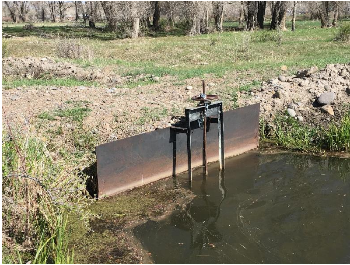
Headgate looking downstream
