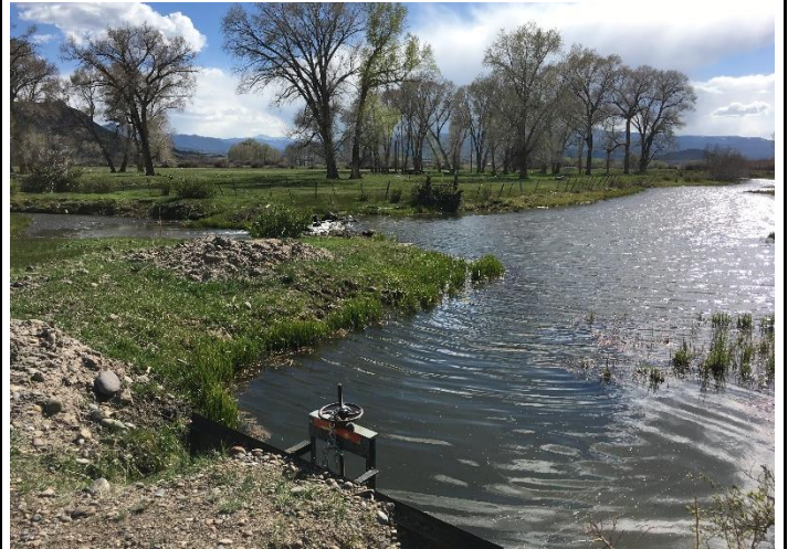
Headgate and diversion dam
