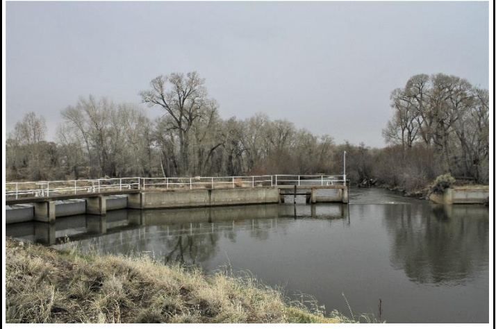
Headgate and diversion dam
