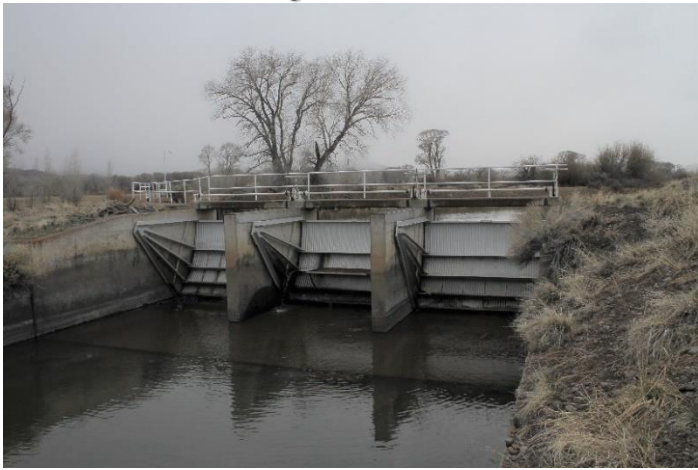
Leaking headgate
