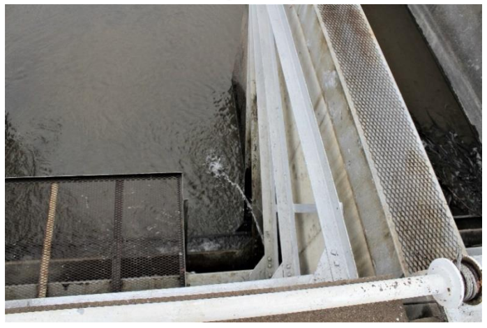
Leaking headgate
