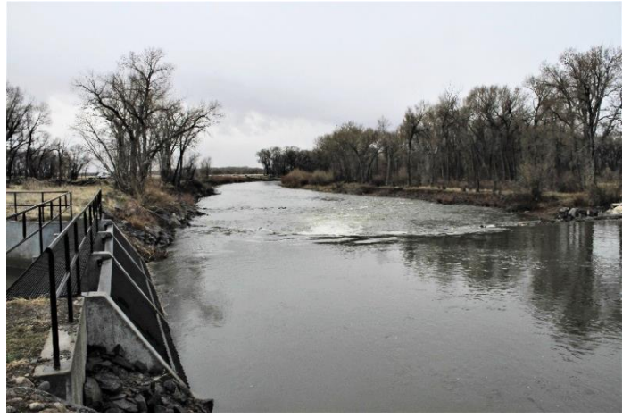
Trash rack and diversion dam
