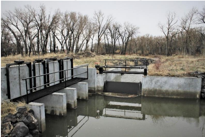
Headgates and sluice gate
