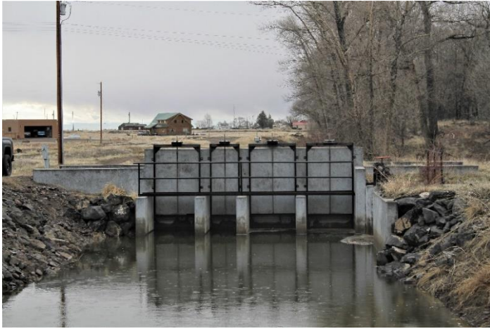
Headgate looking downstream
