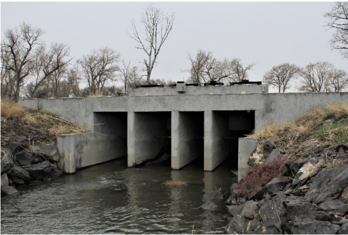
Headgates and sluice gate
