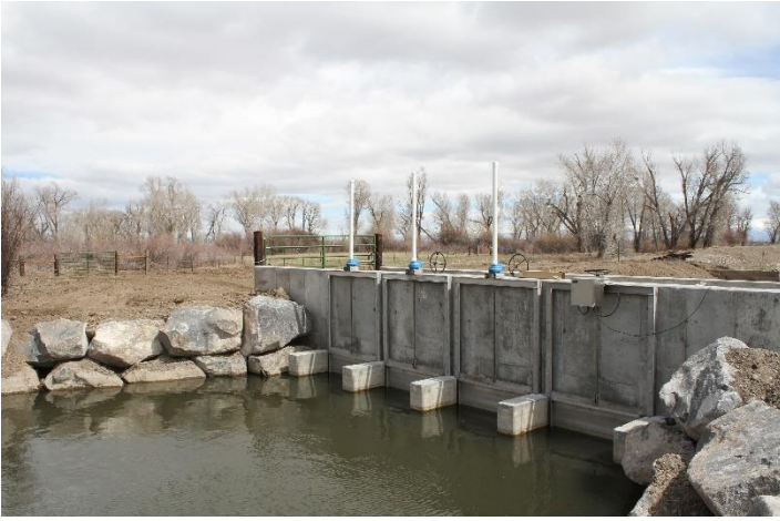
Headgate looking downstream
