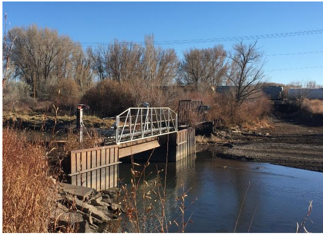
Diversion dam and headgate
