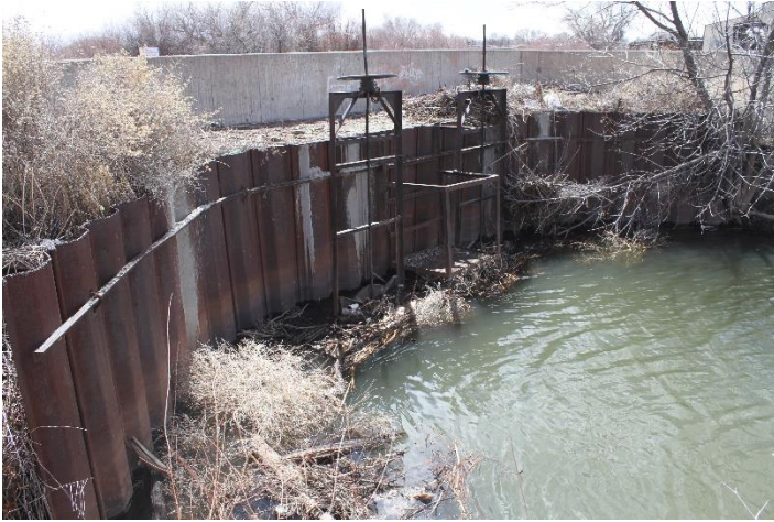
Headgate looking downstream
