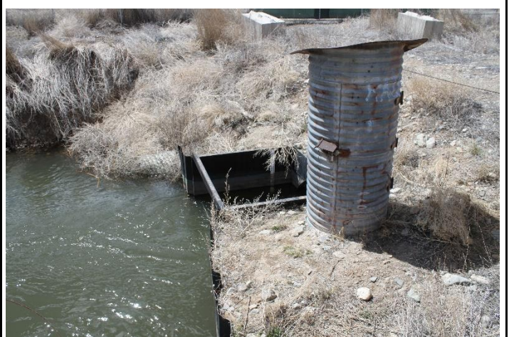
Measurement Structure
