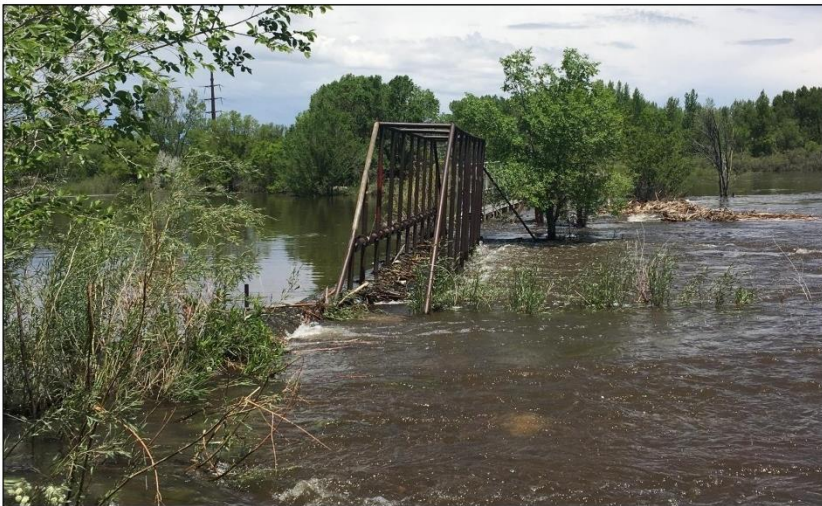
Flooded diversion dam during Spring 2019 runoff.
