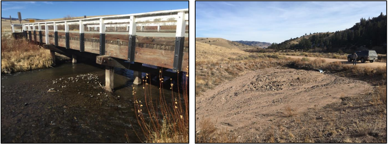
Figure 2.12: (Left) Bridge over Saguache Creek with a pier in the middle of the bridge that may collect debris during a flood. (Right) Undersized culverts failing to transport sediment in a dry wash in Saguache County.
