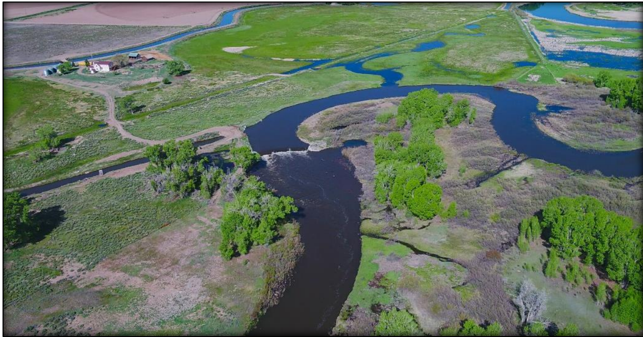
Figure 4.1: Aerial view of the Centennial Ditch diversion (photo: Stuart Penny).
