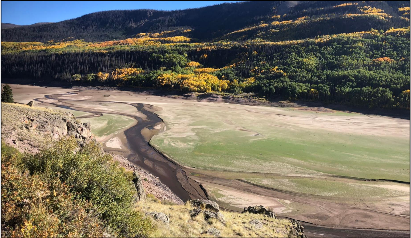
Figure 2.17: Sediment trapped behind the Rio Grande Reservoir (seen during dam repairs which had the reservoir drained during the fall of 2018).
