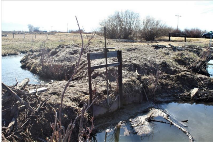
Headgate looking downstream
