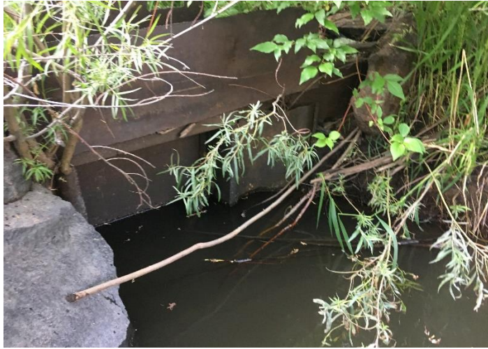
Headgate looking downstream
