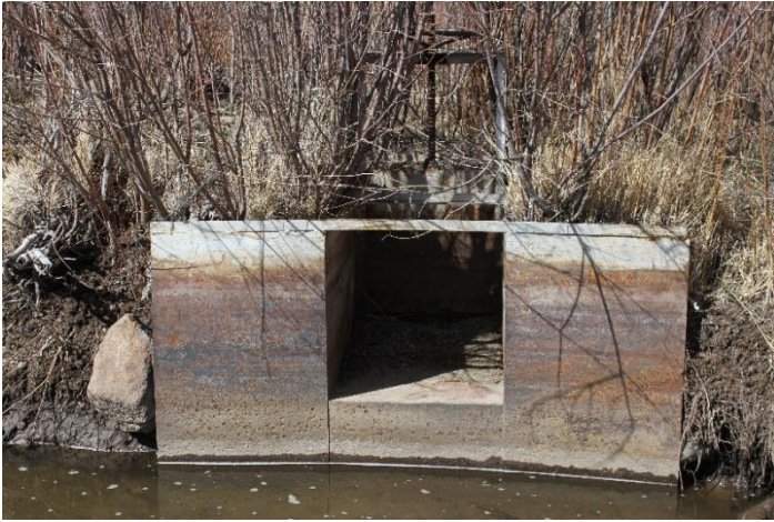
Headgate looking downstream
