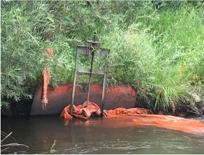
Headgate looking downstream
