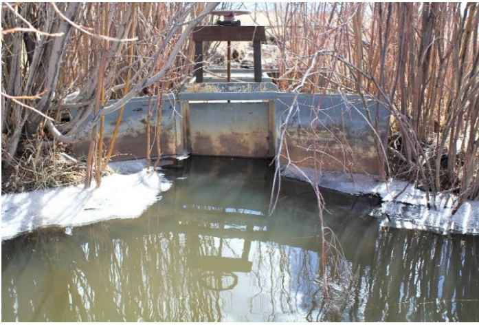
Headgate looking downstream
